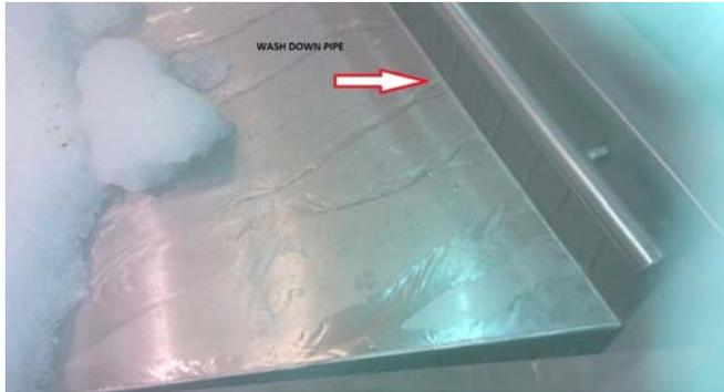
2: Ensure the Drain Grills don't become blocked during wash down. If they block with debris this will lead to water leaking over cabinet.
