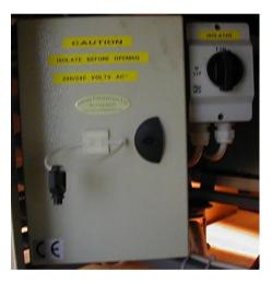
3. This Box contains the PCB Board (Control Unit) also the MCB's which control the power to the compressor, fans, lights and the 13 amp socket located on the punnit end of the Cabinet.
