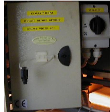
3. This Box contains the PCB Board (Control Unit) also the MCB's which control the power to the controller, fans and lights.
