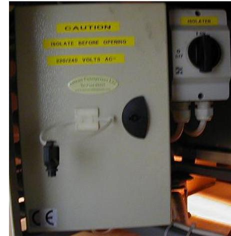
3. This Box contains the PCB Board (Control Unit) also the MCB's which control the power to the compressor, fans, lights and the 13 amp socket located on the punnit end of the Cabinet.
